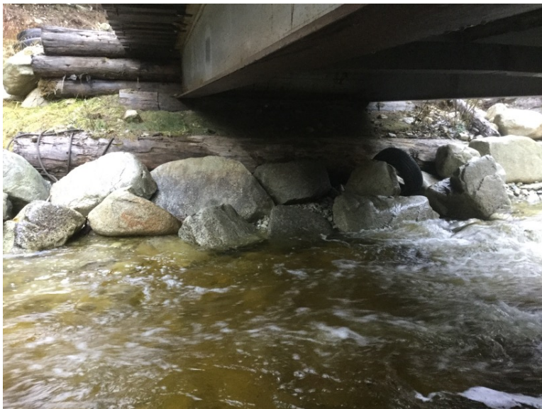
Right Bank Abutment when facing downstream
