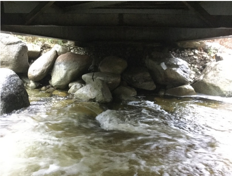
Left Bank Abutment when facing downstream
